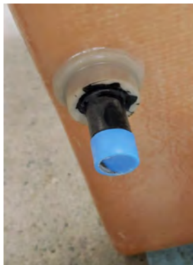
Shown installed from sump exterior
