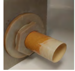
Seat the seal and thread in nut.
