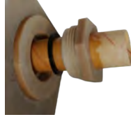
Install seal & nut
