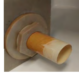
Seat the seal and thread in nut.
