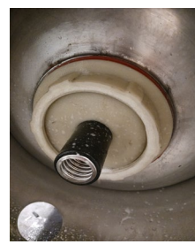
Compression Nut Inside Sump
