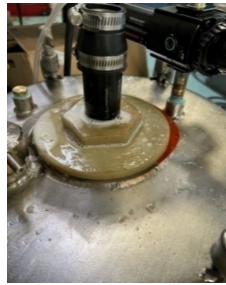
Compression Nut Outside Sump
